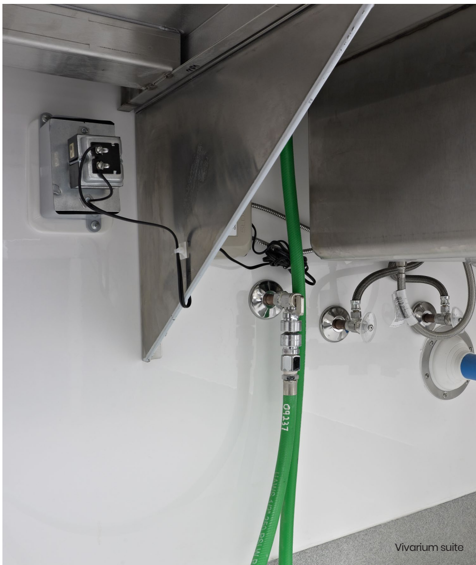
A-1010 Bio-Seal : Quality workmanship is a credit to all involved
