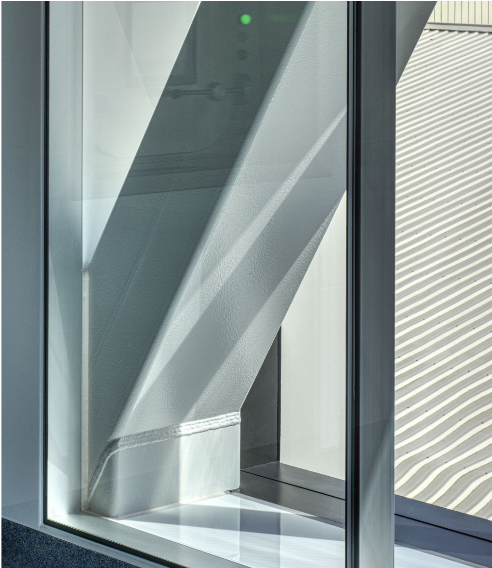
cGMP compliant flush glazed window and fully integrated aluminum extrusion
