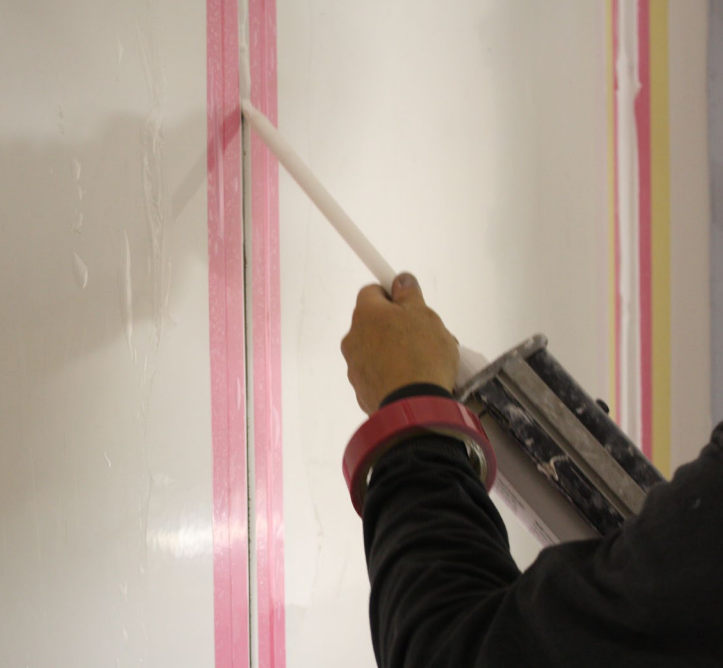
onsite application : A-1010 Bio-Seal three in one - Adhesive Sealant Finishing compound
