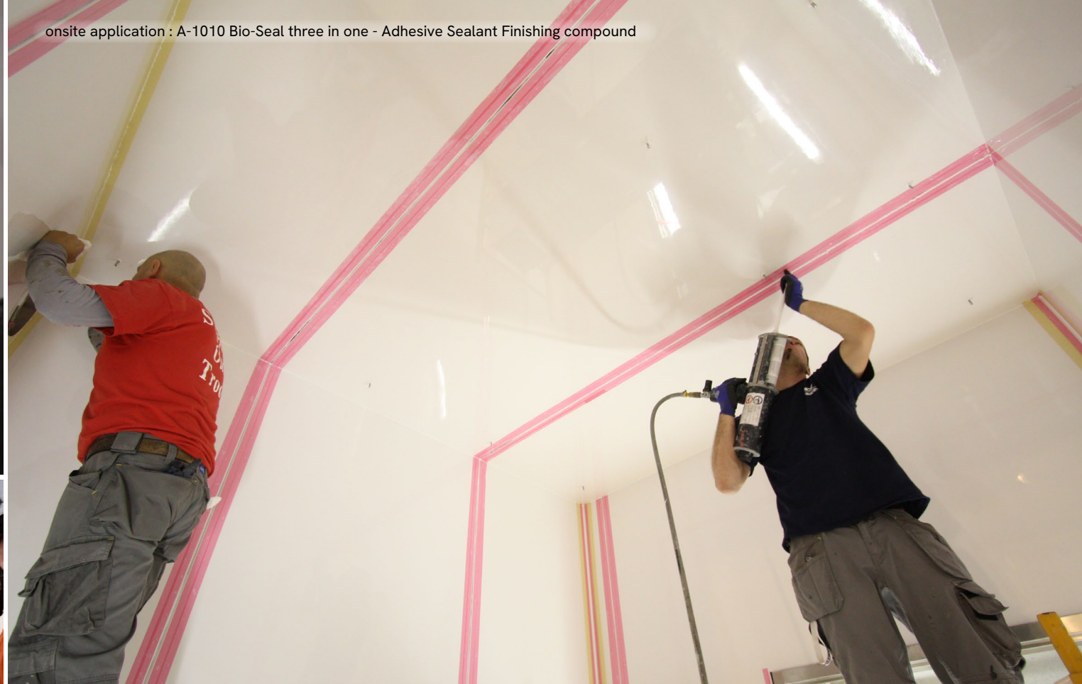
panels are installed with the protective plastic wrapper
